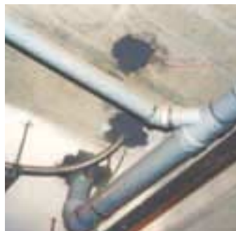
Foam was injected into the vertical pathways to ensure a 100 per cent air seal.
