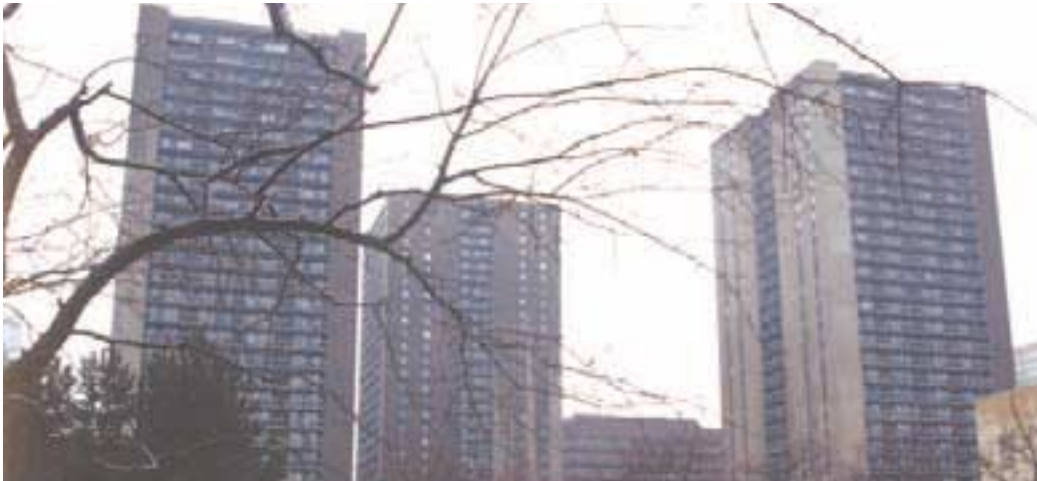
Solving stack effect addressed comfort problems for residents of Forest Laneway and helped save the owners over $200,000 a year in energy bills.
