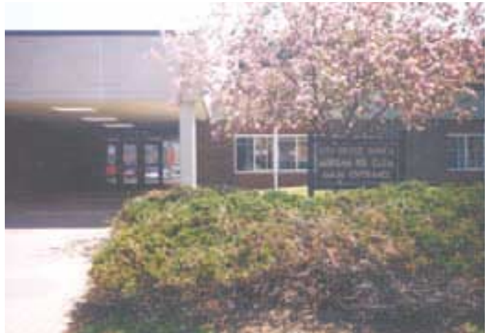
Building envelope repairs performed for the Liverpool Central School District in Metropolitan Syracuse have received positive feedback from teachers and students, as well as other employees.
