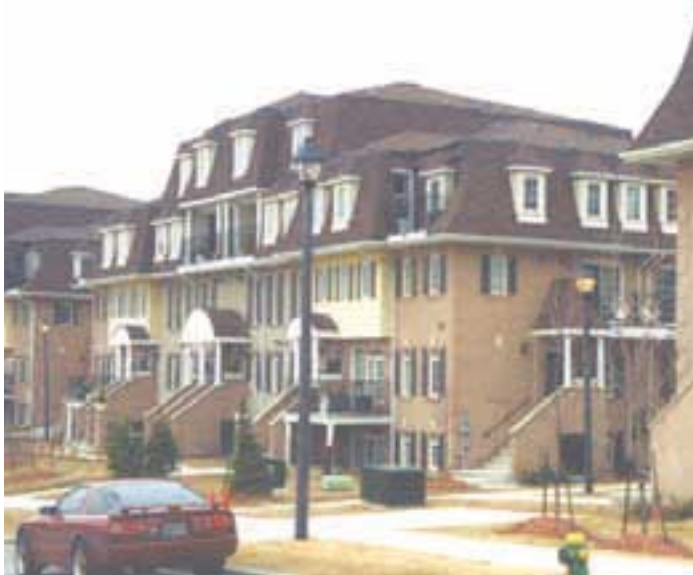
Two-component polyurethane foam was specified by architect Alex Talwood to prevent the migration of exhaust fumes from the underground parking into the units of this Toronto condominium complex.
