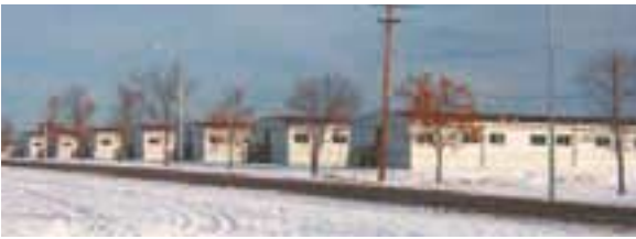
The 134 buildings Canam worked on at CFB Cold Lake include the Maple Flag Quarters.
