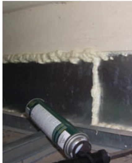
From L to R: overhang surrounding exterior of hospital; site testing; sealing ductwork with ZERODRAFT; pipe penetration leakage site.
