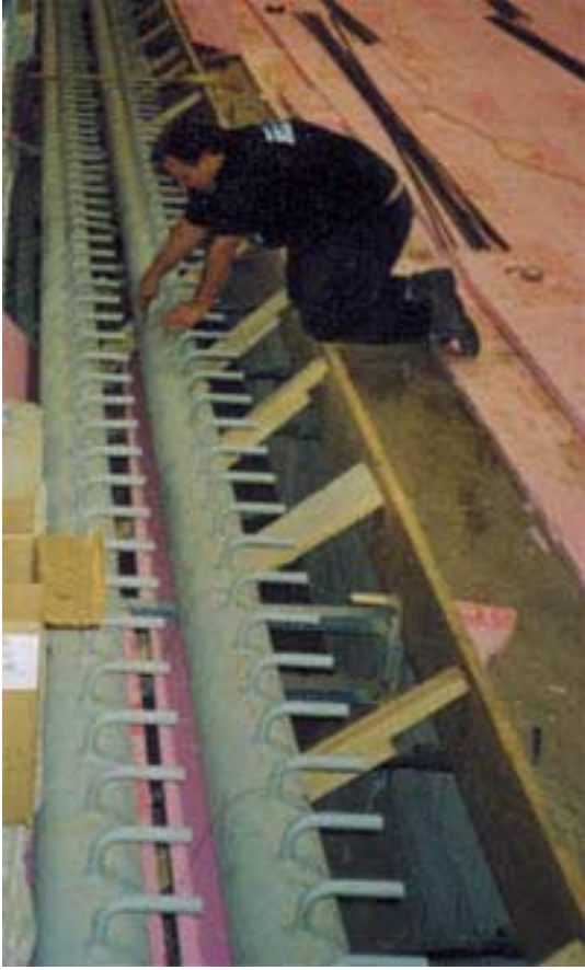
Foam board protects the trench and allows for maintenance access.
